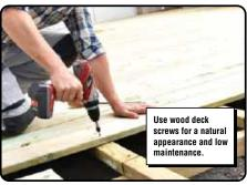
Specially designed for use in wood decking and coated for pressure treated wood.
