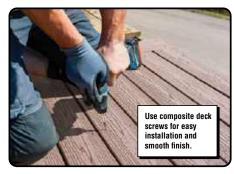
Specially designed for use in composite, or PVC decking.
