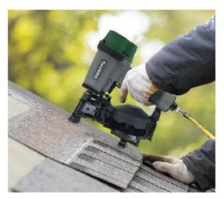
Interchange PRO CR nails are used for asphalt and fiberglass shingles, roofing felt, foam and fiberboard sheathing and installation board.
